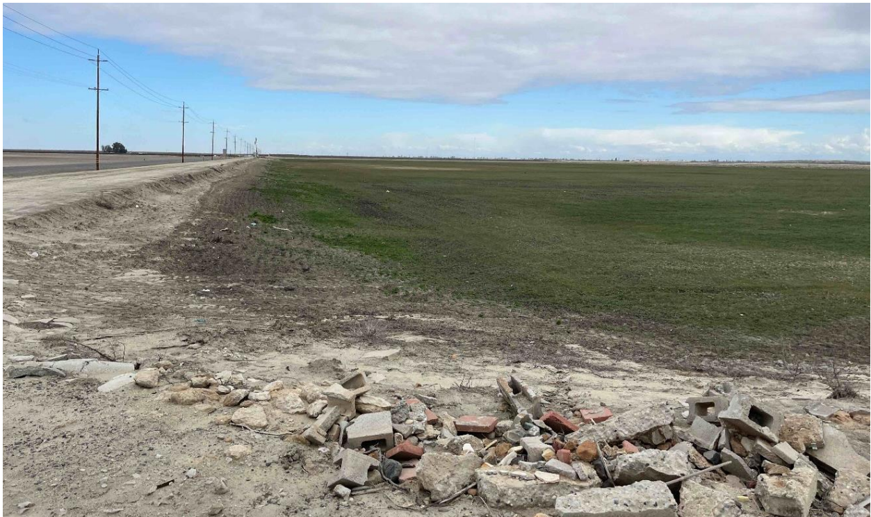
Figure 8 Overview of Canal Debris within Western Site, Facing North
